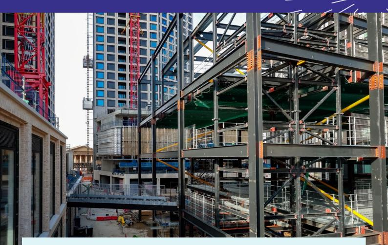
The steel frame for the structure housing some of the retail, leisure and workspace is now complete, paving the way for floor slab installation to commence.
