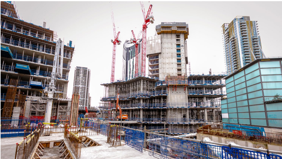
Phase 2 of the main new town centre development.
